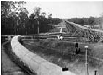
Hudson's temporary scheme, with permanent main under construction
