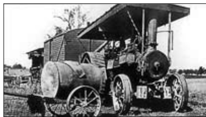
Foden steam traction engine hauling a chaff-cutting plant and cook's galley, Wagga Wagga
