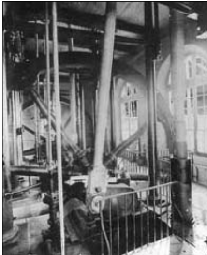
Beam engines at Botany pumping station, installed in 1858
